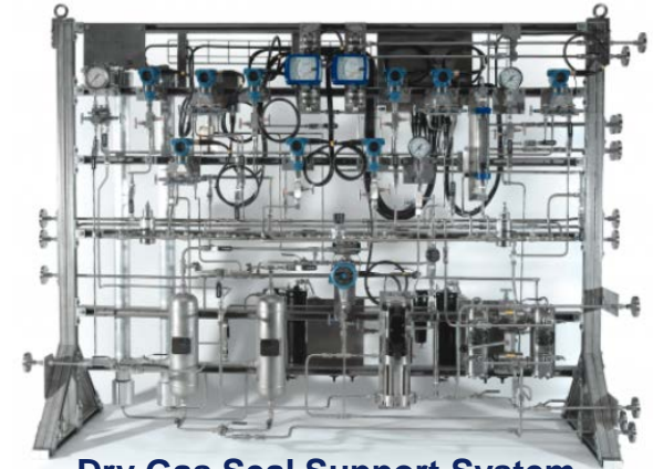
Dry Gas Seal Support System
